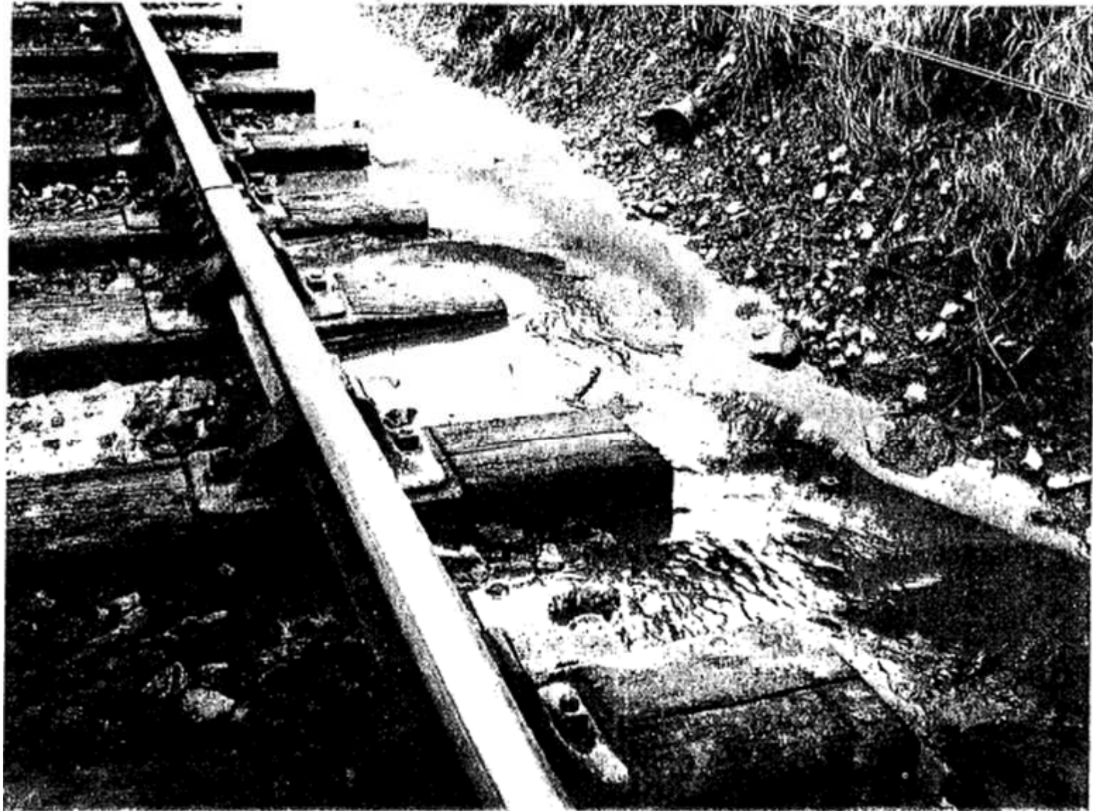
Fig. 9 Pumping of slurry from subgrade attrition
